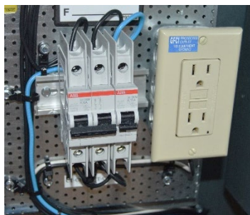
Figure 10: Factory Wired Convenience Outlet
