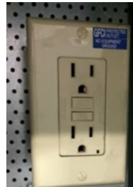
Figure 11: Field Wired Convenience Outlet
