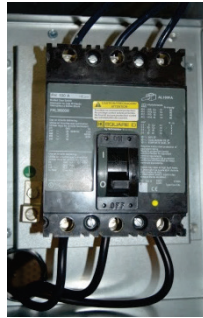
Figure 3 - Non-Fused Disconnect
