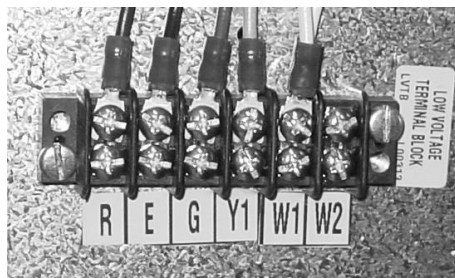
Figure 2 - Example Low Voltage Terminal Block
