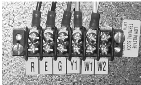
Figure 2 - Low Voltage Terminal Block Example
