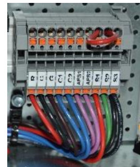
Figure 28 - Example Low Voltage Terminal Block
