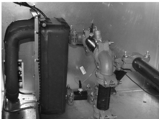
Figure 8 - Insulated Brazed Plate
