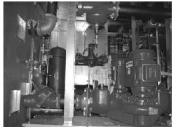
Figure 4 - Chilled Water Pumping Package with dualArm Pump
