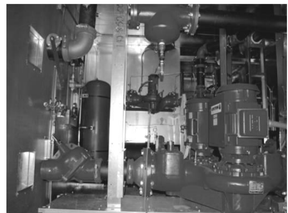
Figure 4 - Chilled Water Pumping Package with DualArm Pump
