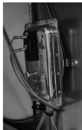
Figure 8 - Clogged Filter Switch
