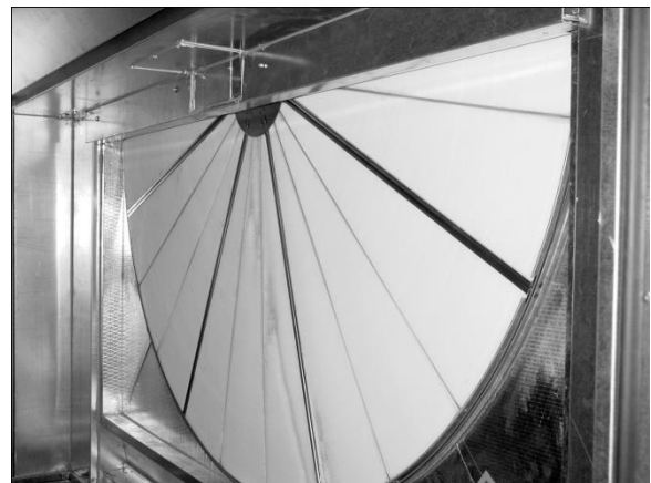
Figure 8 - Energy Recovery Wheel
