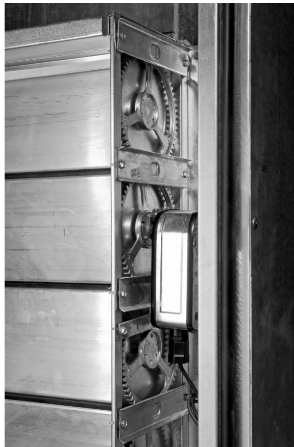
Figure 6 - Gear Driven Dampers
