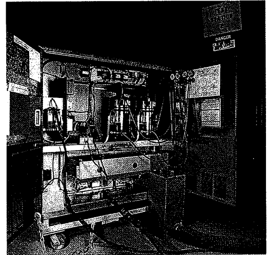
Ready to test
