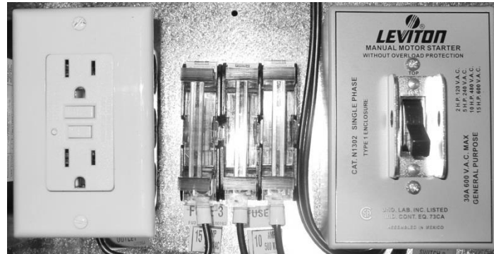
Figure 9 - Factory Wired Convenience Outlet
