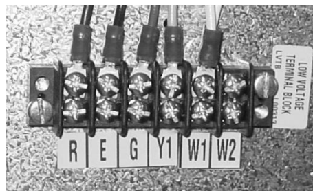
Figure 11 - Example Low Voltage Terminal Block
