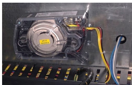
Figure 8 - Supply Air Smoke Detector
