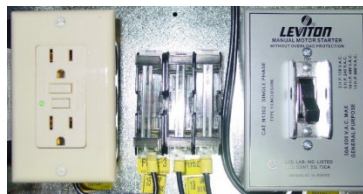
Figure 9 - Factory Wired Convenience Outlet
