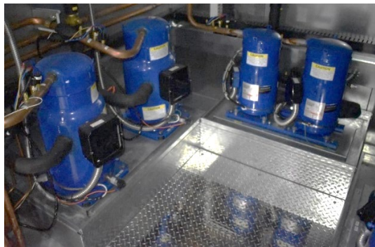
Figure 1 - Variable Speed Scroll Compressor Deck
