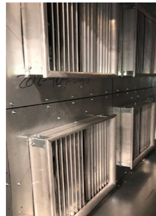
Figure 4 - Inlet Backdraft Dampers
