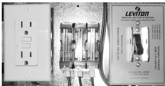
Figure 1 - Factory Wired Convenience Outlet
