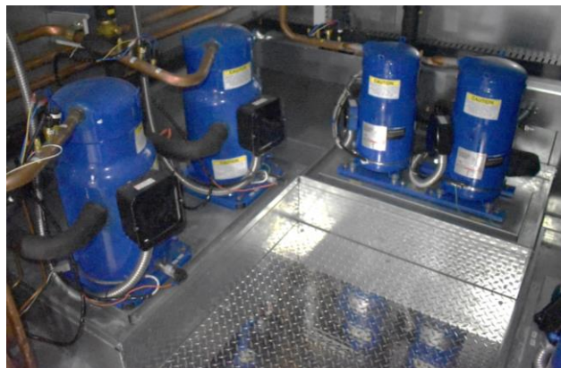
Figure 1 - Variable Speed Scroll Compressor Deck
