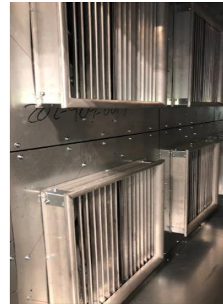
Figure 4 - Inlet Backdraft Dampers
