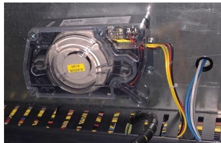
Figure 8 - Supply Air Smoke Detector
