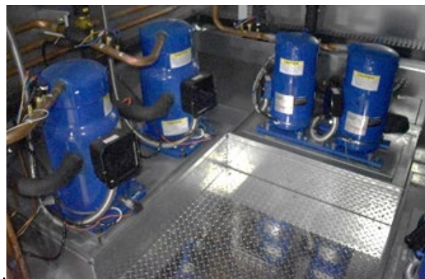
Figure 1: Variable Speed Scroll Compressor Deck
