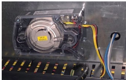
Figure 13: Supply Air Smoke Detector
