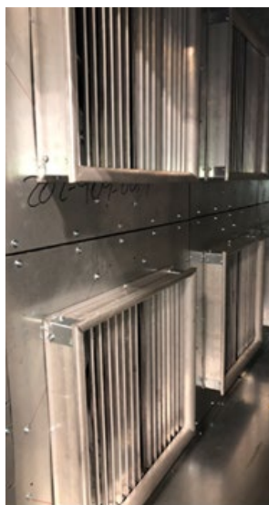
Figure 9: Inlet Backdraft Dampers
