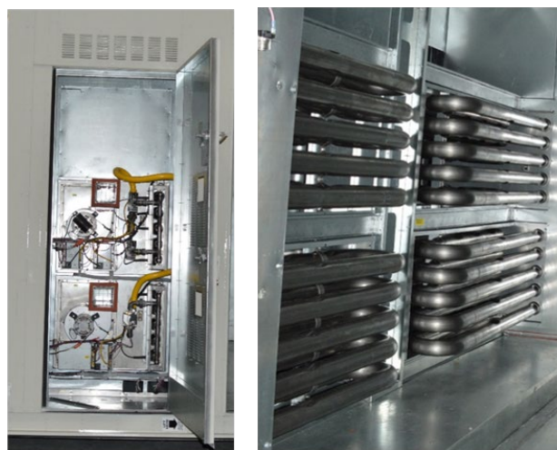
Figure 4: Natural Gas Single Rack Heater
