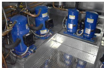
Figure 1 - Variable Speed Scroll Compressor Deck
