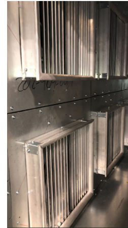
Figure 9 - Inlet Backdraft Dampers
