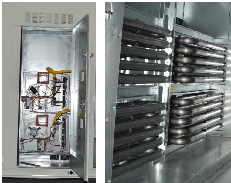
Figure 4 - Natural Gas Single Rack Heater
