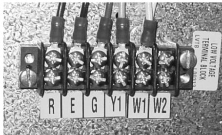
Figure 3 - Example Low Voltage Terminal Block
