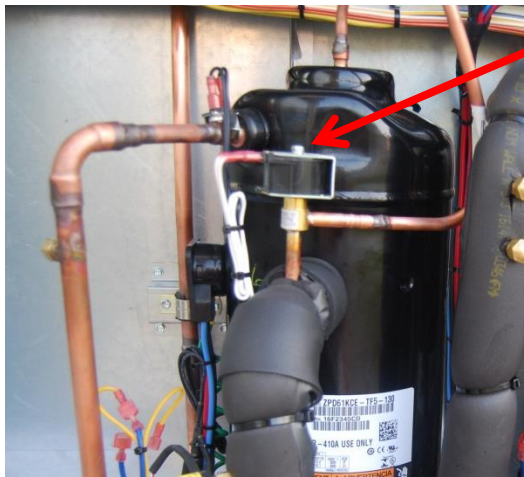
Figure 16 - Digital Compressor Solenoid
