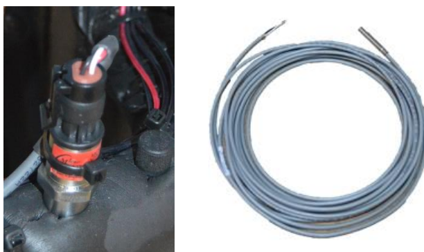
Figure 37 - Suction Line Sensors
