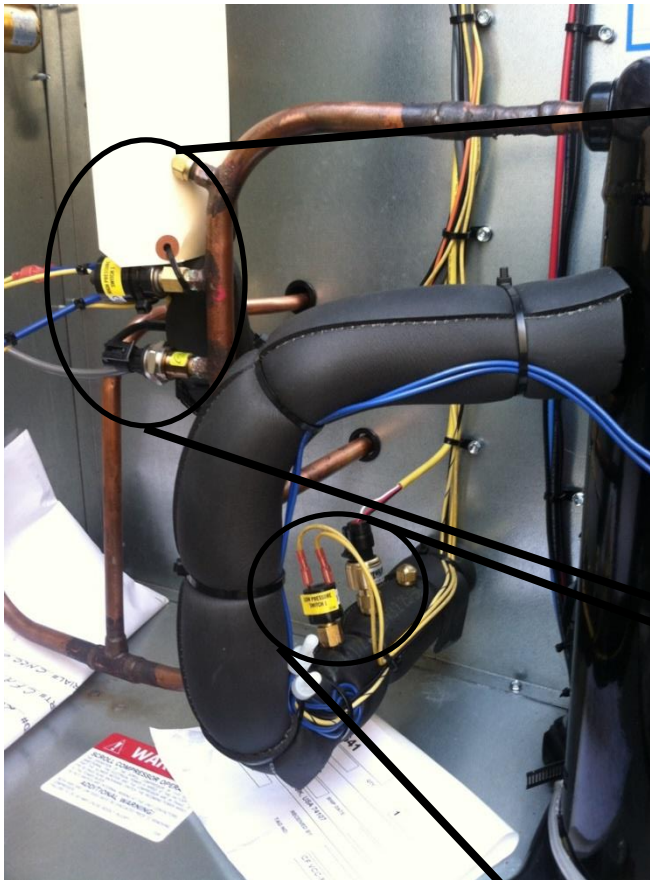
Figure 133 - Schrader Valves Installed on Discharge and Suction Lines
