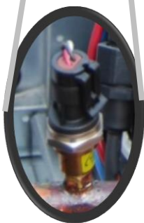
Figure 148 - Discharge Pressure Transducer
