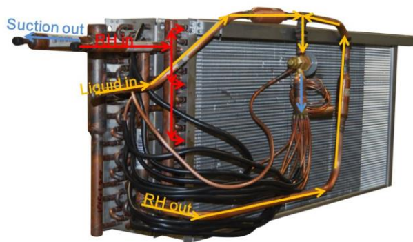
Figure 65 - Reheat Coil in AHU
