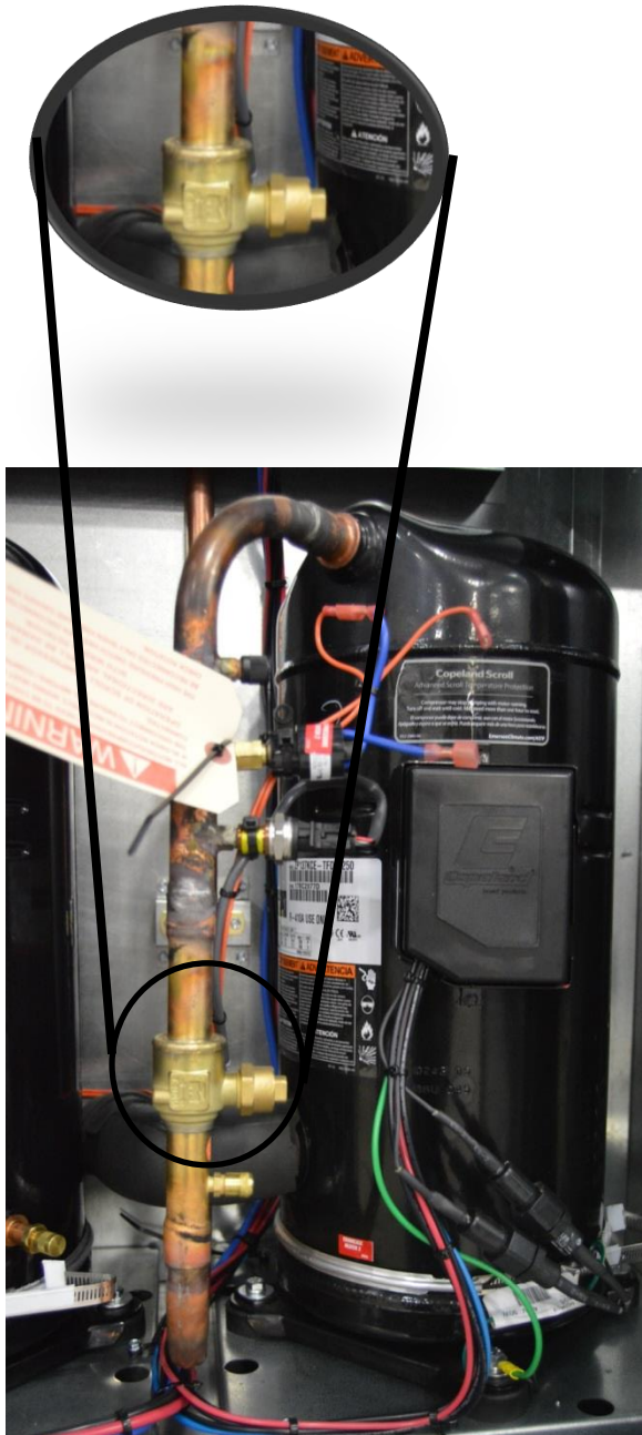
Figure 129 - Compressor Isolation Valve
