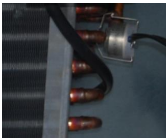
Figure 79 - Freeze-Stat
