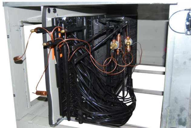
Figure 45 - E-coated DX Coil
