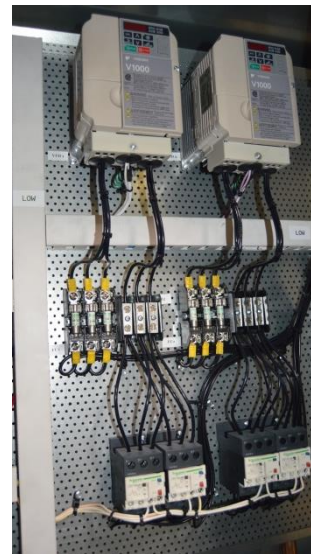
Figure 137 - VFD Controlled Condenser Fan Head Pressure Control
