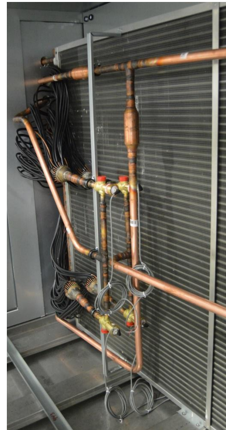
Figure 35 - EXVs in AHU
