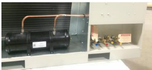
Figure 98 - Horizontal Receiver Installed in Condensing Unit
