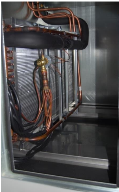
Figure 27 - TXV in Air Handling Unit
