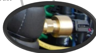
Figure 151 - Suction Pressure Transducer
