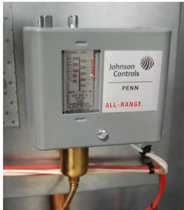
Figure 134 - Adjustable Fan Cycling Switch
