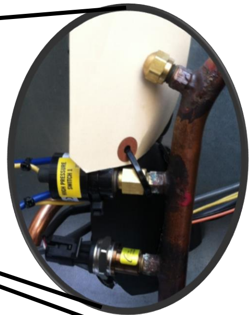
Figure 132 - Schrader Valve
