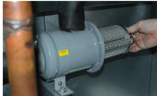
Figure 119 - Suction Line Filter
