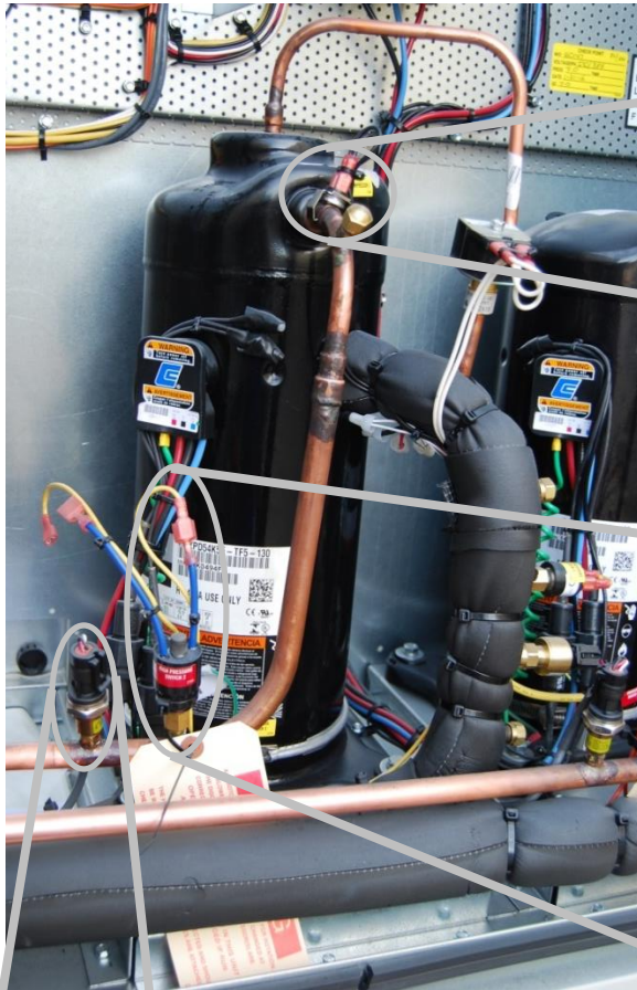
Figure 147 - Digital Discharge Thermistor
