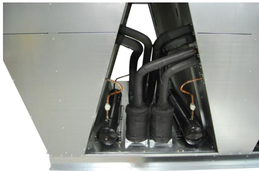
Figure 71 - Air-Source Heat Pump Condensing Unit
