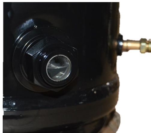
Figure 14 - Compressor Oil Sight Glass & Oil Service Connection
