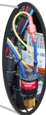
Figure 146 - High Pressure Switch
