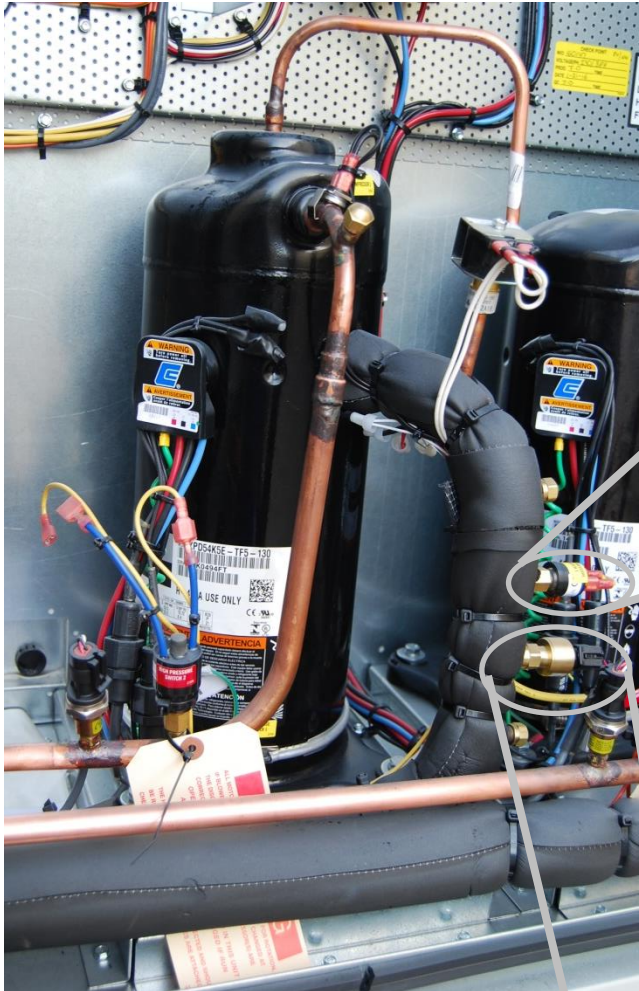
Figure 149 - Digital Compressor Circuit
