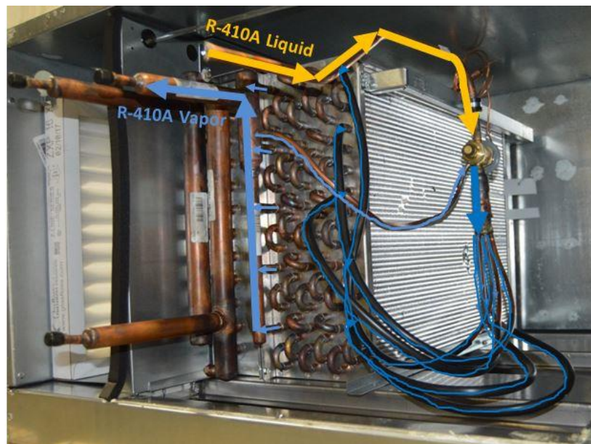
Figure 42 - Refrigerant Flow through a DX Coil
