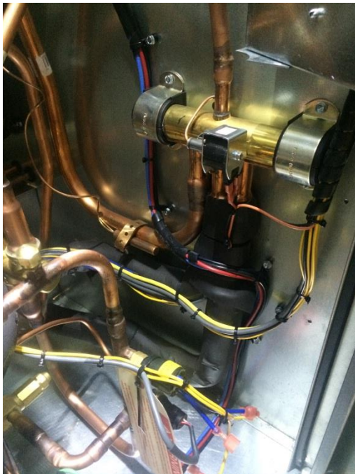
Figure 73 - Reversing Valve Installed in Condensing Unit
