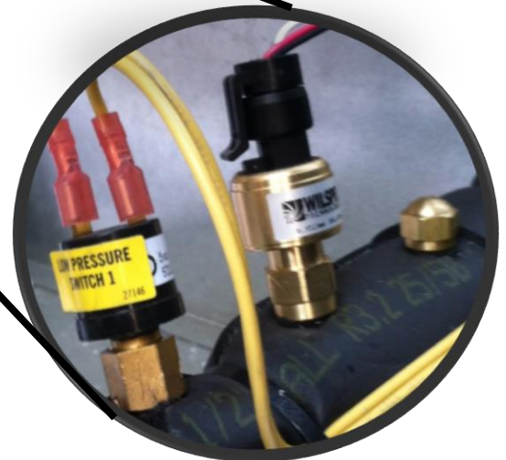
Figure 133 - Schrader Valves Installed on Discharge and Suction Lines
