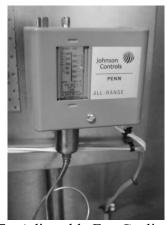
Figure 7 - Adjustable Fan Cycling Switch
