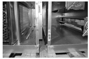
Figure 11 - Connect Sections
