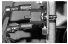
Figure 49 - Rollout Switch
