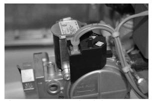
Figure 43 - Gas Control Switch
