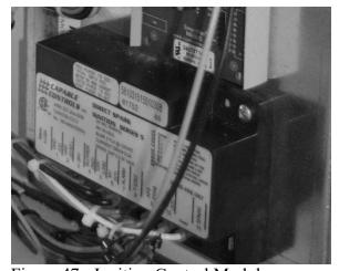
Figure 47 - Ignition Control Module
