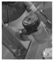
Figure 51 - Condensate Drain Overflow Switch
