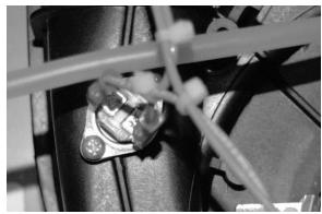
Figure 50 - High Limit Switch on Fan Housing
