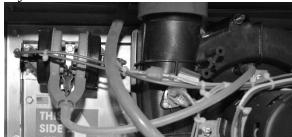
Figure 48 - Air Pressure Switch for two-speed draft inducer
