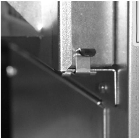
Figure 8 - Filter Rack Closed with Clip
