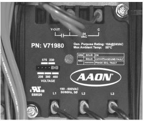
Phase and brownout module may be this type on some products (as seen in the above picture). No setup is needed with this module version, other than checking that the voltage jumper voltage matches the unit voltage
