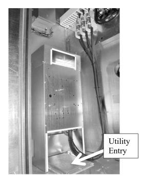
Figure 8 - Back View of Utility Entry and Power Switch from Control Compartment (75-140 ton Units)
