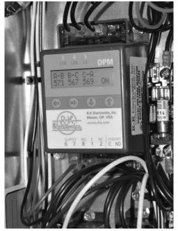
The DPM is a Digital Phase Monitor that monitors line voltages from 200VAC to 240VAC 1φ and 200VAC to 600VAC 3φ. The DPM is 50/60 Hz self-sensing. DPM must be wired according to unit specific wiring diagram include in the control compartment
