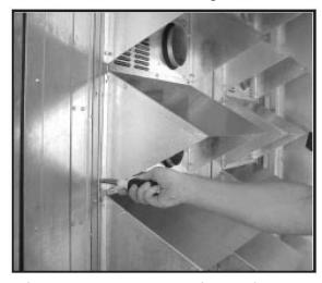
Figure 39 - Gas Heater Rain Hood Screws
