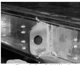
Figure 3 - Base Rail Lifting Lug
