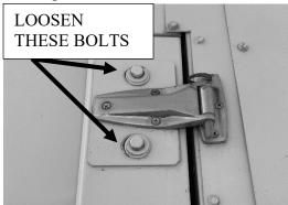
Figure 33 - Evaporative condenser access door
