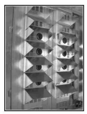
Figure 38 - Gas Heater Rain Hood
