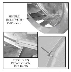
Figure 22 - Securing the Band
