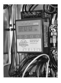
The DPM is a Digital Phase Monitor that monitors line voltages from 200VAC to 240VAC 1¢ and 200VAC to 600VAC 3¢. The DPM is 50/60 Hz self-sensing. DPM must be wired according to unit specific wiring diagram include in the control compartment
