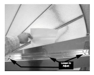
If it is necessary to adjust a purge seal to the face of the wheel, loosen the two or three screws along the bearing beam and adjust to the proper distance from the media surface. Tighten the screws and retest the seal.
