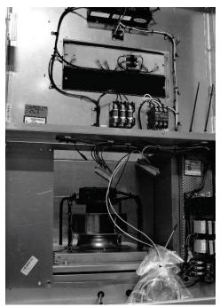
Figure 5 - Supply Fan Access after removing control panel
