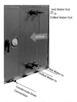
Figure 23- Hot & Chilled Water Piping
